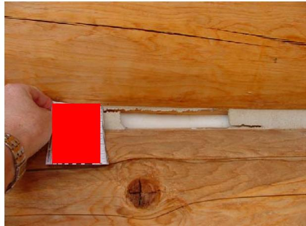
*Figure 5. - Adhesively failed chinking at wood-to-wood log joinery.*
