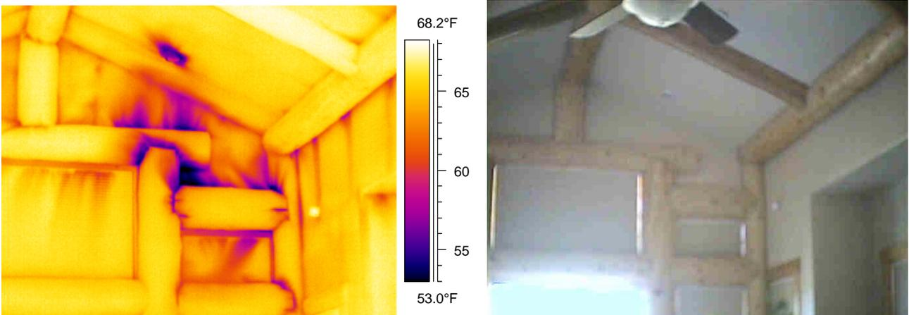
*Figure 7 & 8. – Extensive air infiltration during depressurization at numerous wood-to-wood joinery locations where logs are exposed on interior of wall. Reference scale for temperature differential of 15.2°F between 68.2°F and 53.0°F.*
