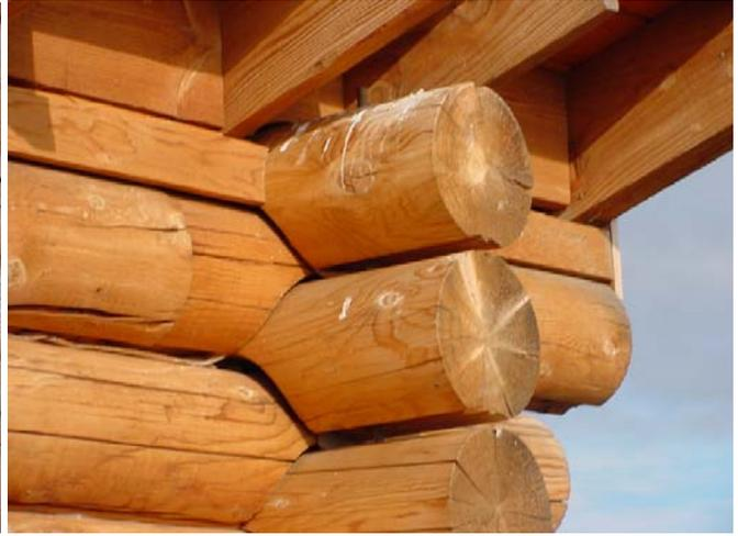
*Figure 3. Open / un-sealed butt joint between logs.*
