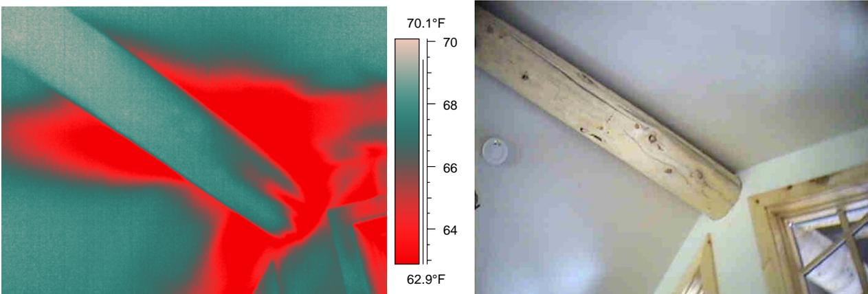
*Figure 21 & 22. - Large cooling area clearly illustrates extent of air infiltration at top of beam where access is difficult and closure/sealing may have been altogether left out.*
