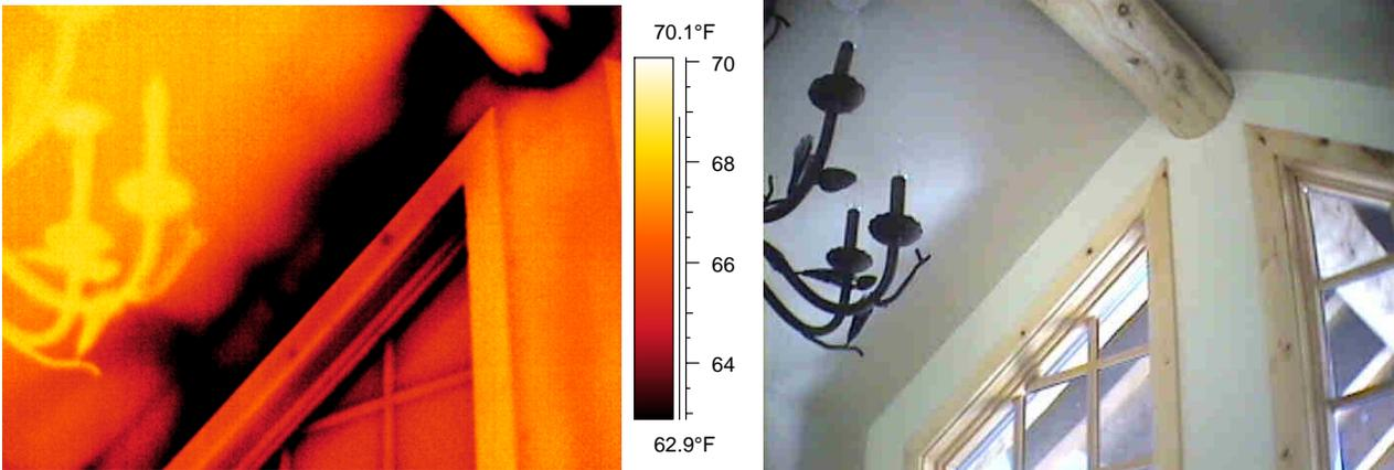
*Figure 19 & 20. - Infrared cameras reveal substantial cooling during depressurization both around the ridge beam log and also at the sloped interface between the drywall and vaulted ceiling. Note that large openings existed between the log wall and roof soffit immediately opposite this image. These openings were permitting substantial air infiltration.*
