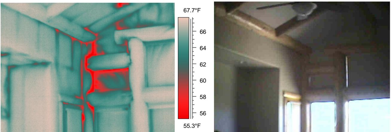
*Figure 9 & 10. - Extensive air infiltration at wood-to-wood joinery in log assembly.*
