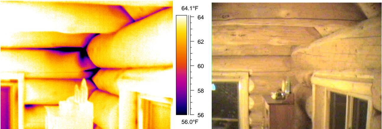
*Figure 15 & 16. – Cooling patterns at corner joinery which extends at horizontal joints in log.*
