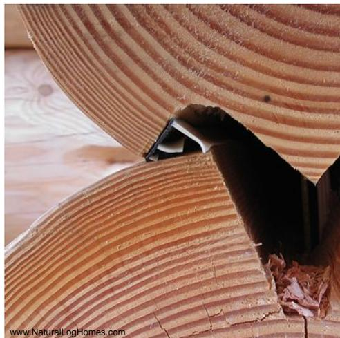
Here, in a window opening, you can see our gasket's 3 white fins, short, medium and long, and how they point down to, and seal against, the log below. The black rubber base is stiffer than the first fins. The gasket is stapled to the upper log only through the black base, and only in the gaps between the fins.
