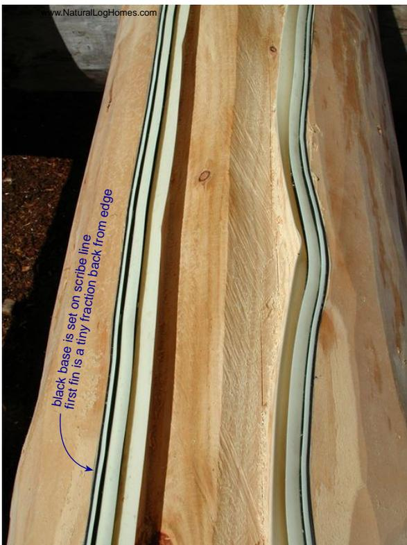
The NLH gasket is soft enough to conform to curved shapes of groove edges. The 3 fins point down to the surface of the log below, and provide 6 barriers to air infiltration when installed as shown in this photo. Also note the tiny fraction of black rubber base that goes right on the scribe line -- the first, shortest, white fin is just back from the gasket edge.
