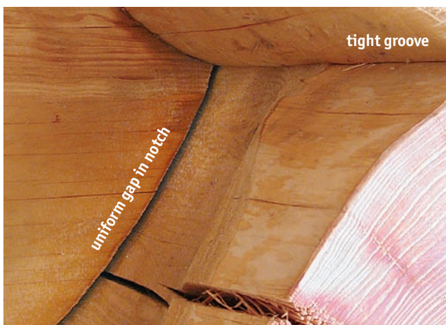
Figure 2: This building was not underscribed. As the logs dried, the long grooves stayed tight, while corner notches got gaps. The even width of the notch gaps prove that the scribing and cutting was carefully done: the gaps are not from poor craftsmanship, they're from normal and expected shrinkage. Underscribing solves this problem—underscribing helps keep the notches tight over time.
