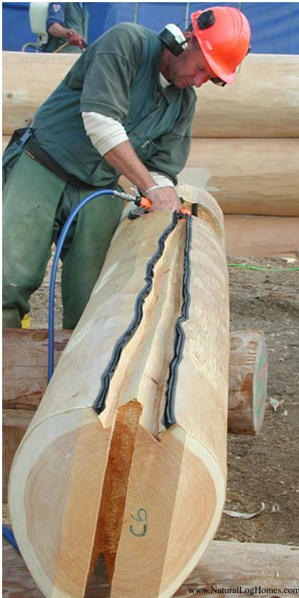
Installing the gasket into the long groove with a pneumatic stapler. One man can install about 150 lineal feet of gasket per hour-- that's 20 hours total for a typical 3-bedroom log house, with 2 layers of gasket in grooves and all notches, as shown.
