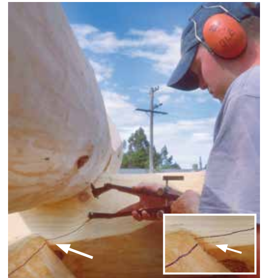
Figure 3: The groove was scribed, then the scribers were closed down slightly, and now Olaf is scribing the notch. The notch scribe line is a little above the groove scribe line—the difference in height is the underscribe amount.
