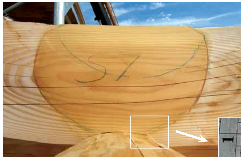
Figure 6.b: In the building yard, about 100% of the weight of the building is on the notches, and very little weight is on the grooves. In this photo you can see that the notch has compressed the saddle, and this is the result that we want.
