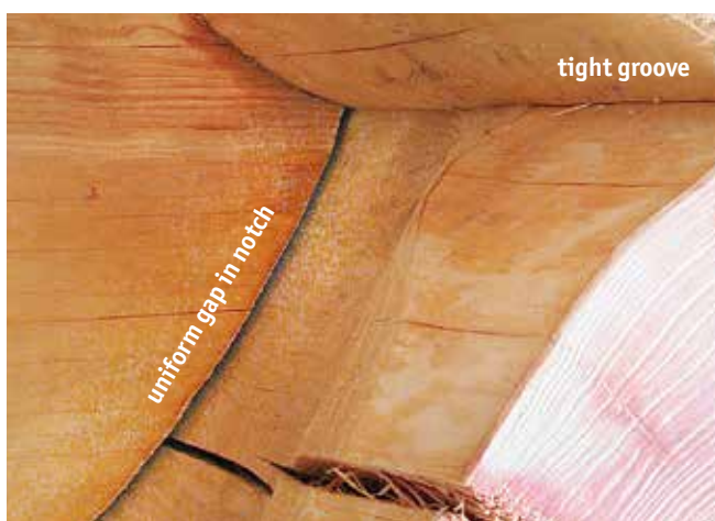
Figure 2: This building was not underscribed. As logs the logs dried, the long grooves stayed tight, while corner notches got gaps. The even width of the notch gaps prove that the scribing and cutting was carefully done: the gaps are not from poor craftsmanship, they're from normal and expected shrinkage. Underscribing solves this problem—underscribing helps keep the notches tight over time.
