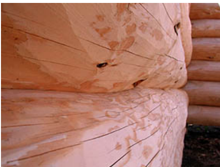
The scribed fits are the same quality as one-log-at-a-time log fits. This close-up photo is from a 2004 Natural Log Homes Accelerated project.
