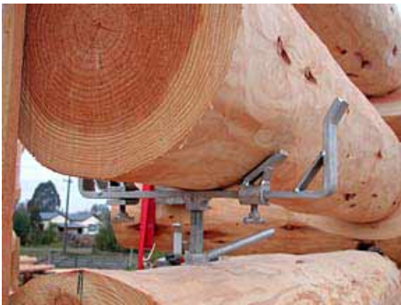
A "goal post" holds a one-notch log in the stack.
