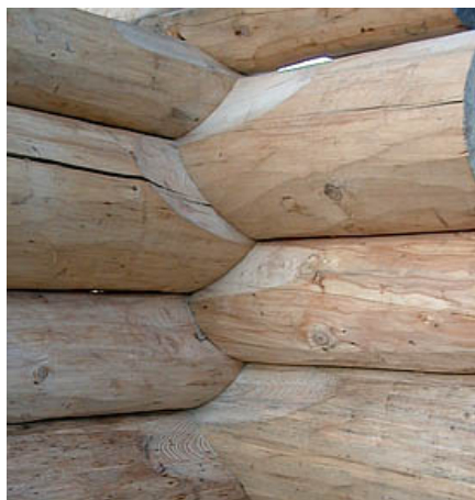
"After" — the same corner after cutting. To get your bearings and compare it to the "before" picture, note the checked log in the upper left of each picture.
