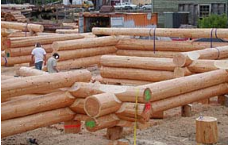
"One Log At A Time" at Natural Log Homes in 2003. Each log must be fully, finally fitted before a "next log" can be added to any wall.
