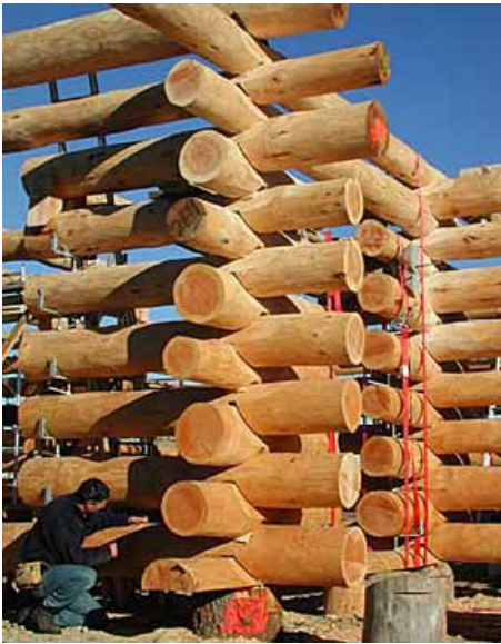
This NLH Accelerated stacked shell is ready to scribe.
