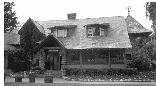
Figure 6: A classic with low pitch roofs, eyebrow shed dormers; gable dormers, a tower with kicked hips; and a broken-back valley (on far left). The variety of roof planes and styles really makes this building interesting. It has charm and pleasing proportions—a human scale that is naturally welcoming, cozy, and appealing.
