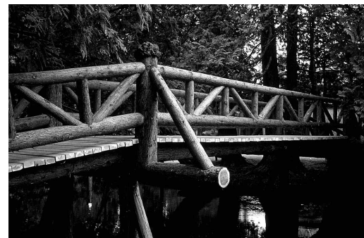
Figure 5: Adirondack-style footbridge made of scribe-fitted white cedar poles with the bark left on.
