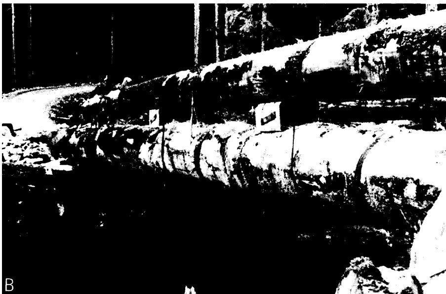
Figure 1.—Log stringer bridges. A—large log stringers are simply placed on log crib abutement. B—bridge with spread brow logs; this bridge spans nearly 100 feet and is designed for 80-ton off highway logging trucks. (M 143 536) (M 143 751-16)
