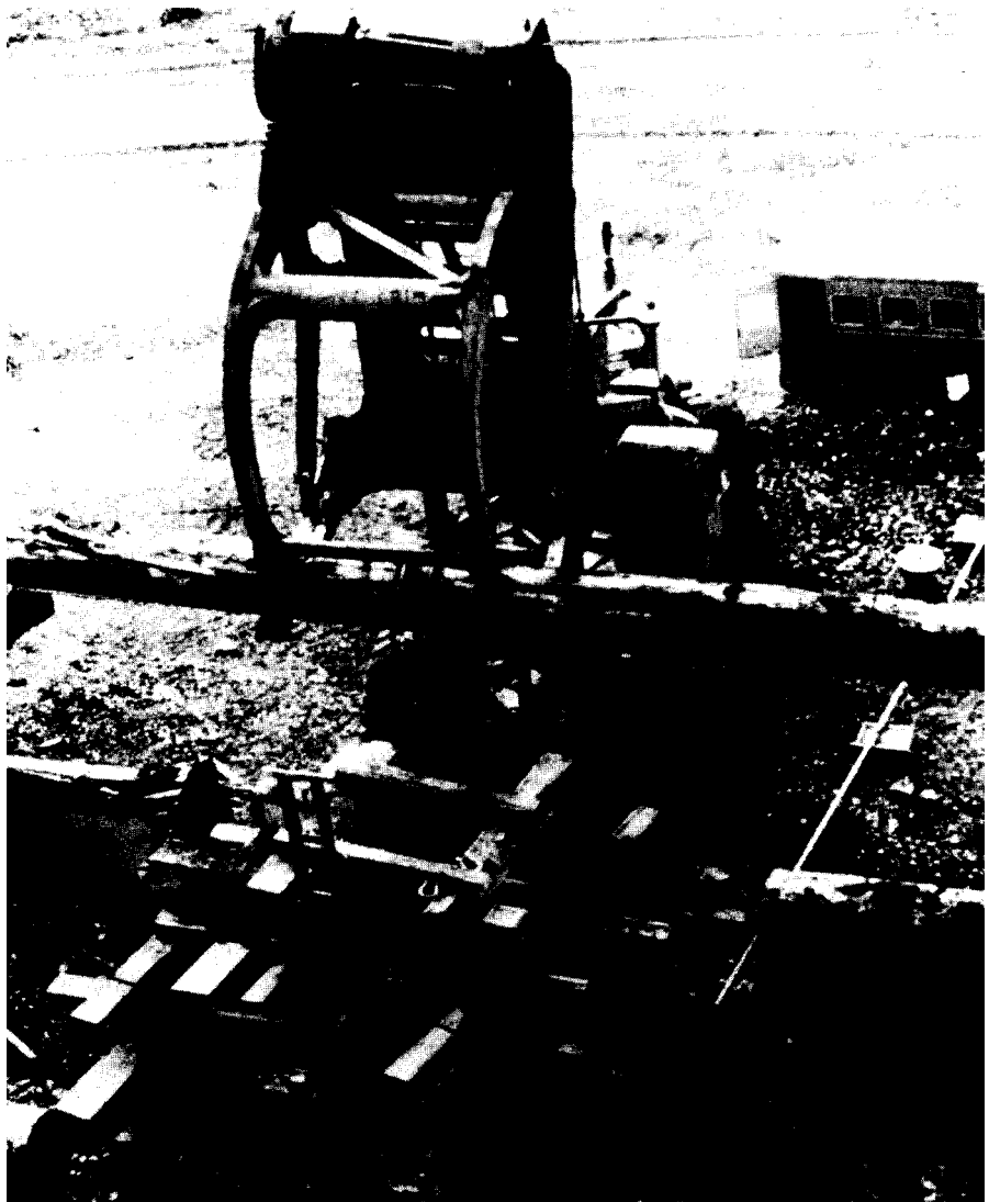
Figure 10.—Giant log stacker placing test log up on supports. Logs had to be lifted approximately 20 feet. (M 143 750-13)
