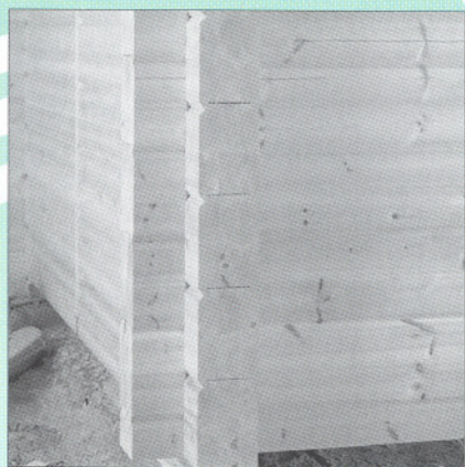
Figure 4. A log intersection
