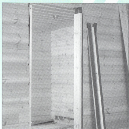
Figure 7. A tongued jamb in a door opening
